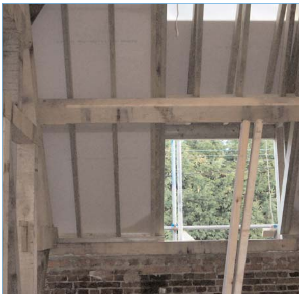
SUPALUX® – unaffected by rain during construction
