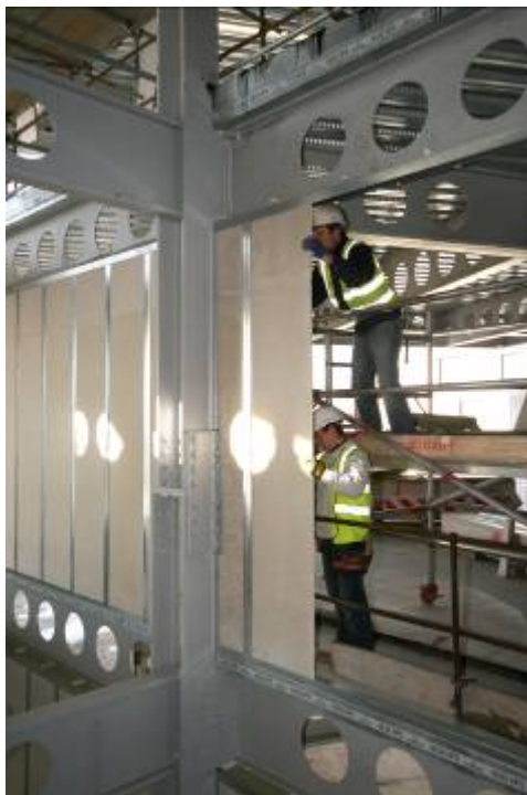
Promat SUPALUX ® Shaftwall system provides up to 120 minutes fire protection
