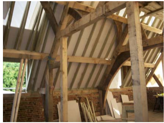
Promat SUPALUX® THATCH with the fair face exposed to the building interior
