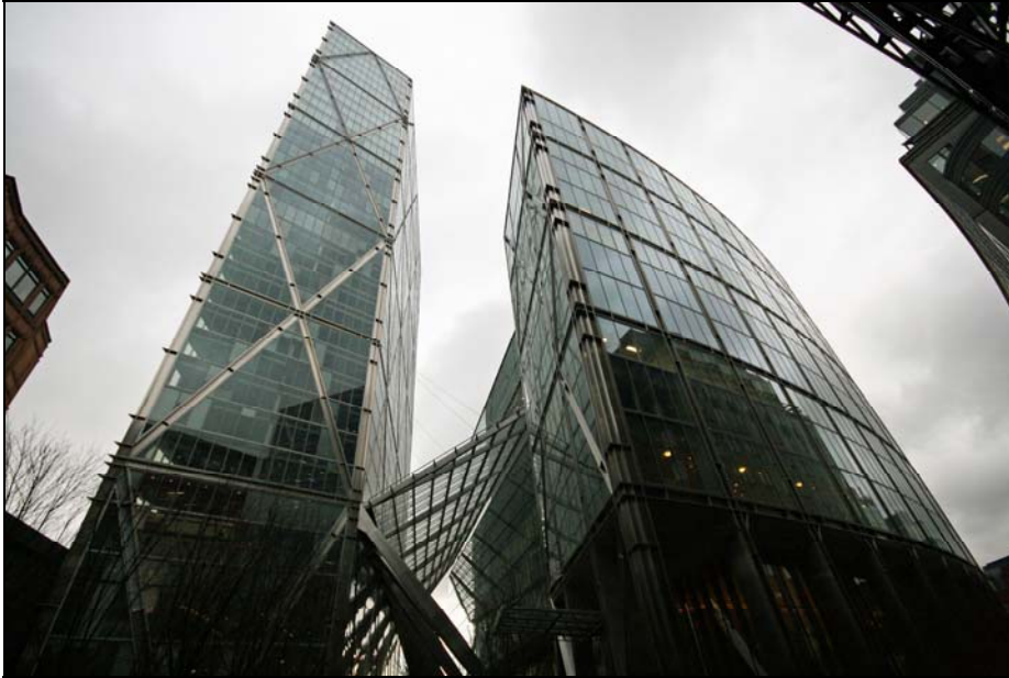
Broadgate Tower and 201 Bishopsgate: the largest ever speculative office development undertaken in London
