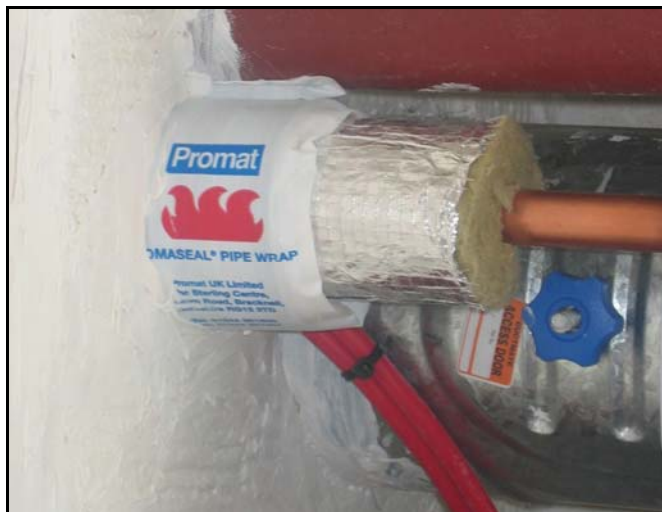
Promat PROMASEAL® range of Fire Stopping products prevent the spread of fire, smoke and toxic gases through service penetrations.
