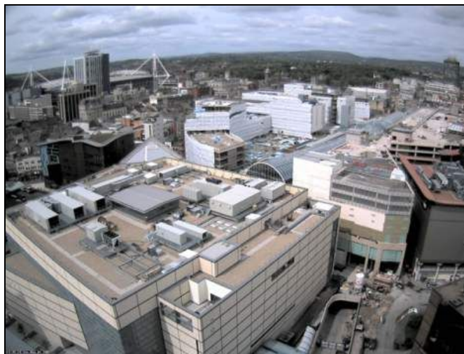
CAPTION: Promat has supplied fire protection solutions to 'St David's 2' development in Cardiff
