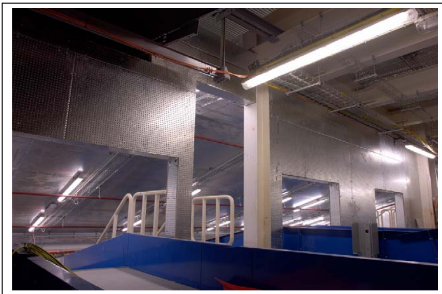
Pic 3: Passive fire protection methods control the spread of a fire, buy time for a building's occupants to escape, help fire fighters tackle the blaze and also limit the damage wherever possible.
