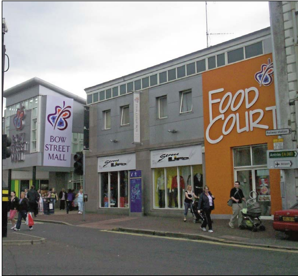
Promat SUPALUX providing Fire Protection to Bow Street Mall, Lisburn
