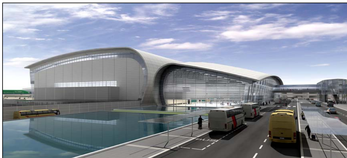
Promat UK has supplied fire protection solutions for Dublin Airport's new Terminal 2 building
