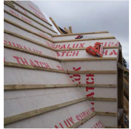
Promat SUPALUX® THATCH creating complete roffing envelope.
