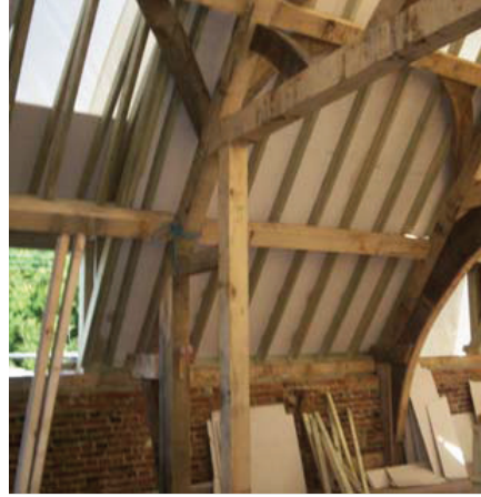
Promat SUPALUX® THATCH with the fair face exposed to the building interior.
