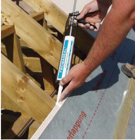
The use of Promat PROMASEAL® Intumescent Acrylic Sealant.
